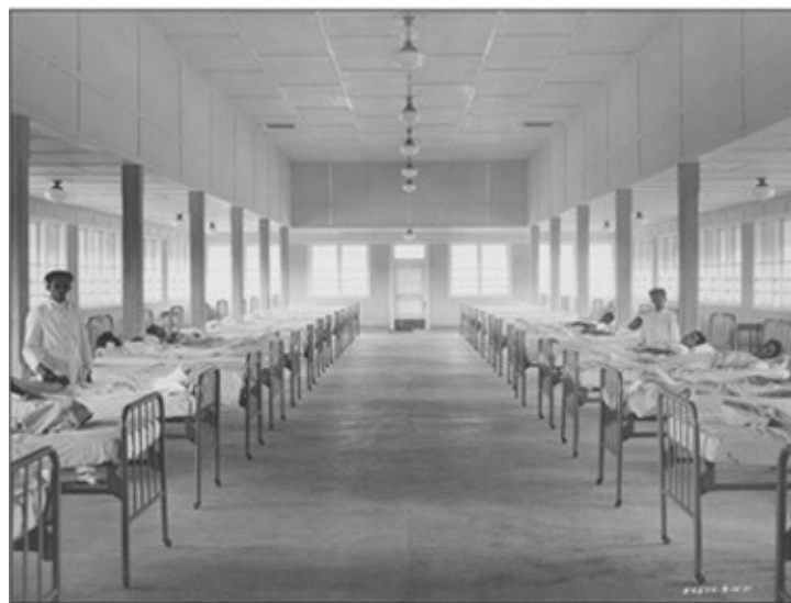
Top: An “ambulance” arrives at Fordlandia’s hospital, designed by Albert Kahn. Below: The scene in the hospital ward.
