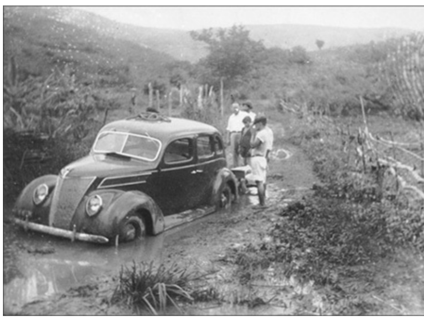
New roads to roam: A Lincoln Zephyr stuck in Fordlandia mud.
